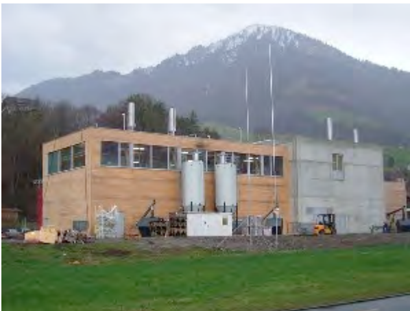
Figure 5: View of Nidwalden plant with gasifiers in the left (wooden) building, bunker and peak heaters in the concrete building
